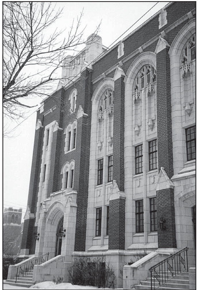
Exterior of Freemasons' Hall, Edmonton, 1998
