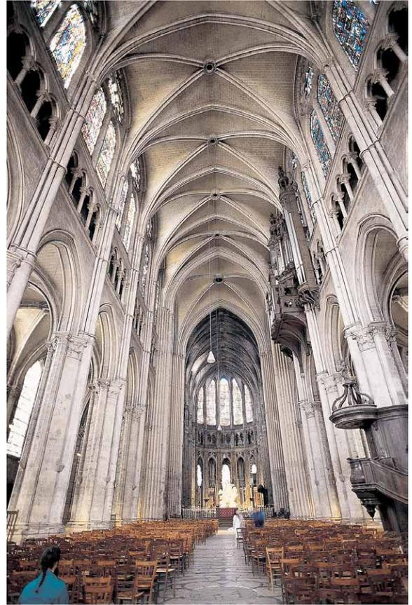
*The Nave of Chartres Cathedral. The flying buttress construction allows the walls to be opened up, flooding the interior with natural light.*
