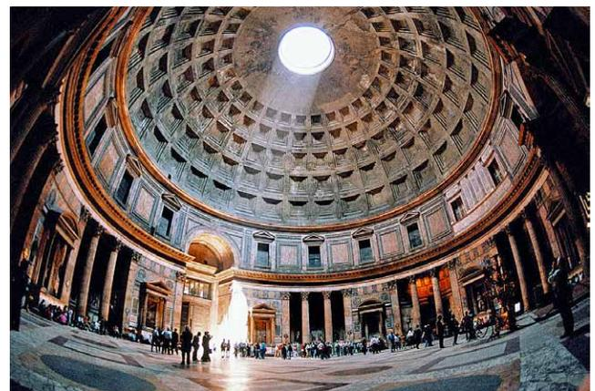
*The dome of the Pantheon in Rome. The coffered concrete dome has an oculus or opening to the sky to let in sunlight. Like a sundial, it illuminates different parts of the interior as the day passes while the rest of the space remains in relative darkness.*
